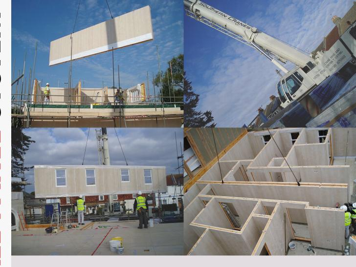
STREIF now offers the widest range of closed and advanced wall panels in the offsite timber frame industry, combining German engineering with British design.
