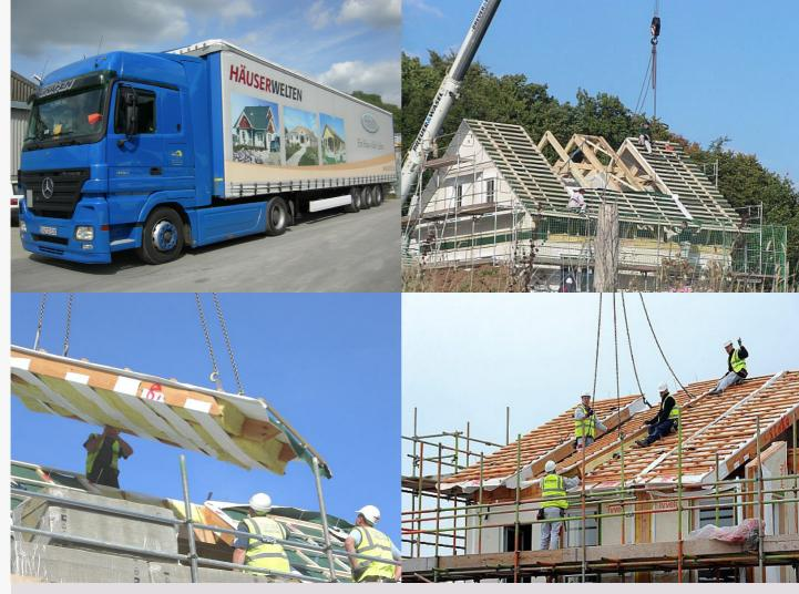
STREIF's heavy duty roof cassette system is the ideal solution for mono pitched roofs, flat roofs and rooms in the roof, when buildings need to be made watertight fast.
