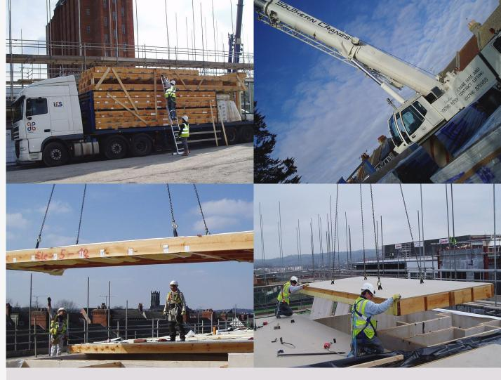
STREIF's heavy duty floor cassette system now provides an attractive alternative to lightweight timber or heavy concrete systems in upper storey floor construction.
